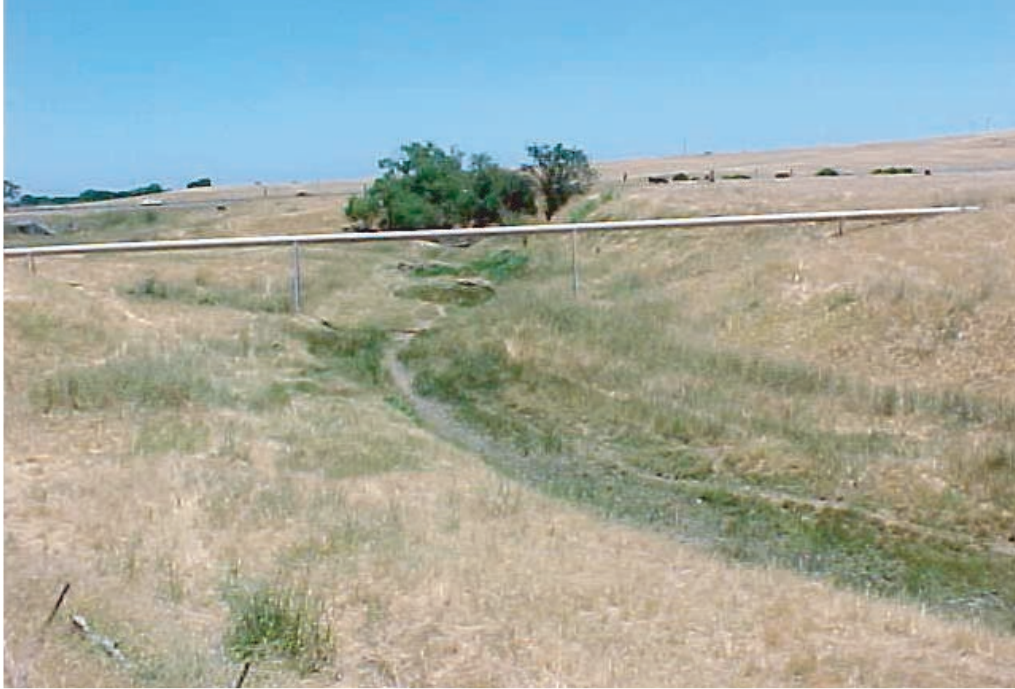
View of degraded channel caused by cattle use
