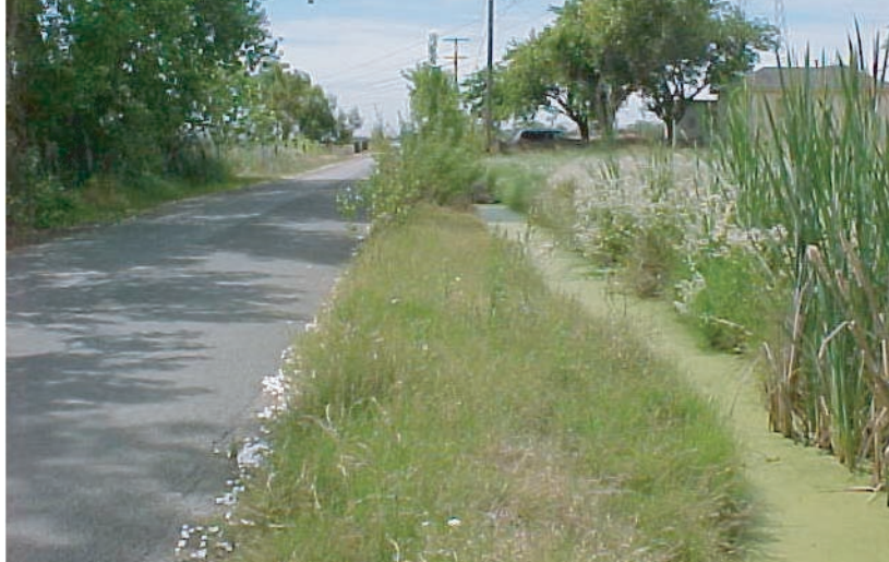
View at roadside drainage ditch near Dutch Slough
