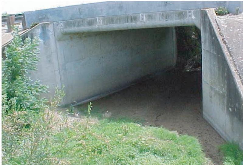
Large box culvert on Lower Marsh Creek at Concord Avenue
