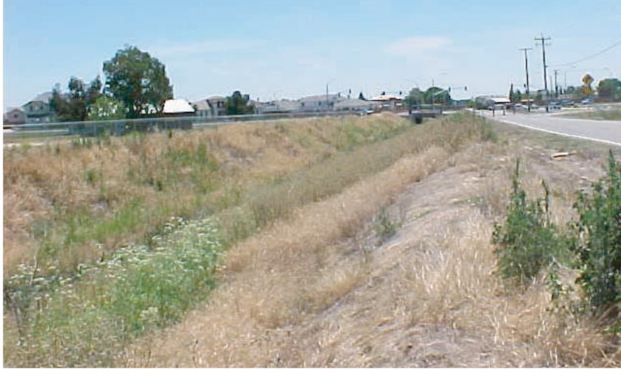
Vegetated flood control drainage ditch
