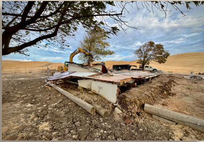
Vaquero Farms Residence Demolition. EBRPD
