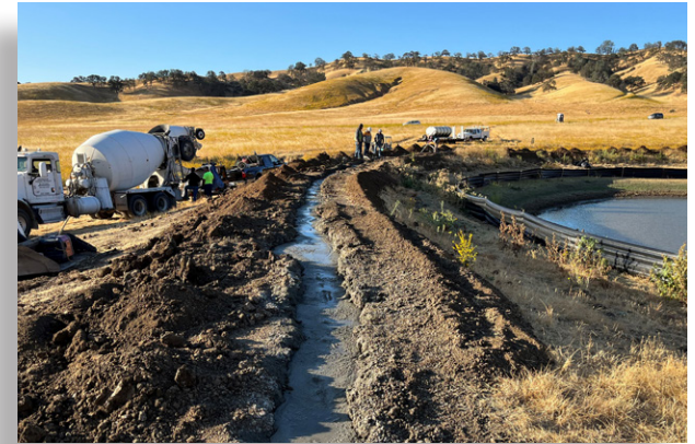
Pond berm repair.
