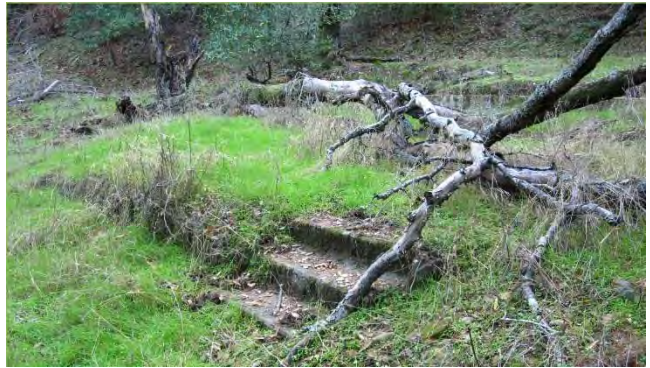
Photo 4: Remnants of the building foundation of the recreational cabin that burned down in the 1970s.
