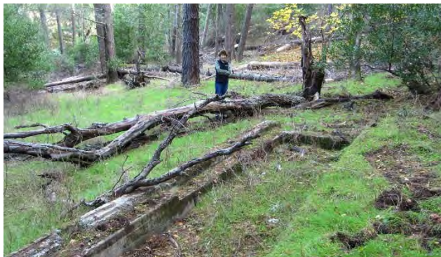
Photo 5: East Bay Regional Park District staff and remnants of the building foundation.
