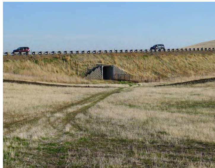
Photo 4: Tunnel under Vasco Road
