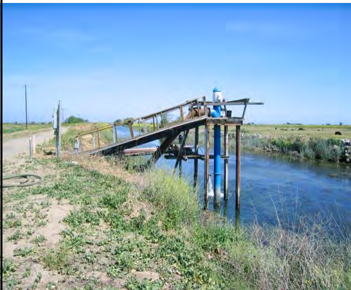
Photo 3: No Name Slough and pump, Southern boundary of the property
