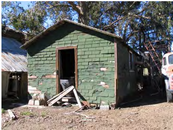
Old Structures at Homestead
